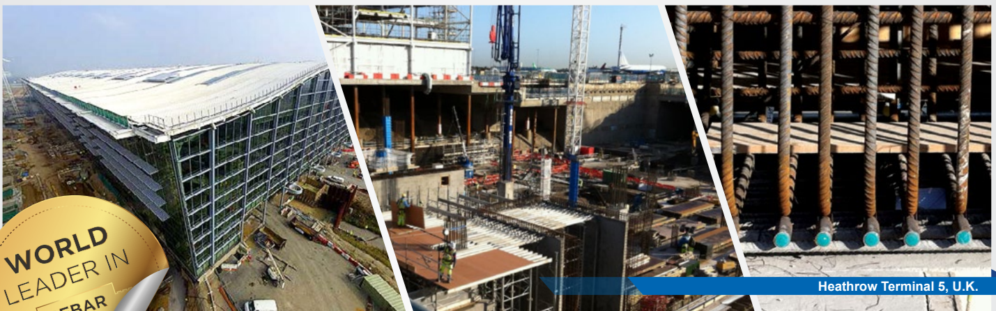
Flamanville nuclear power plant EPR 3, France
